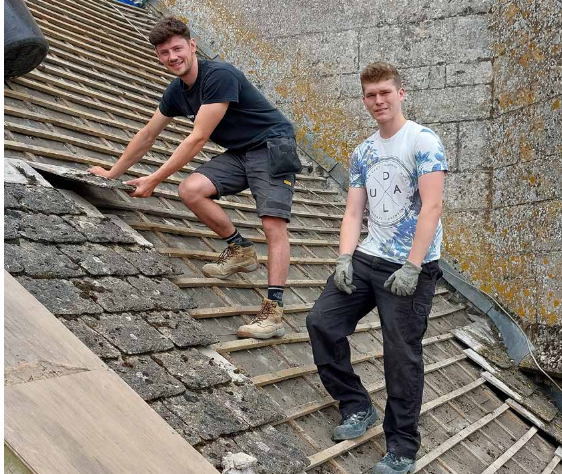
▲ Roofer, Lewis Dowdeswell, with his colleague, Kenzie Stephens, stripping the north nave slope
