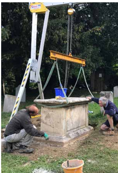
▲ A lifting gantry in use on a table tomb
