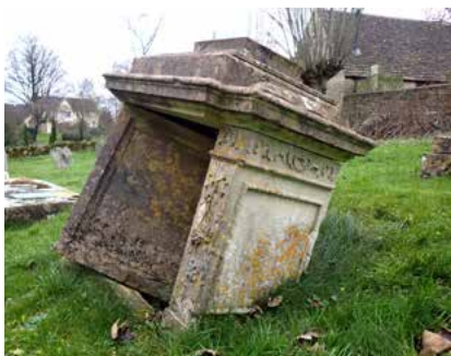
▲ An unstable tomb is an obvious safety hazard
